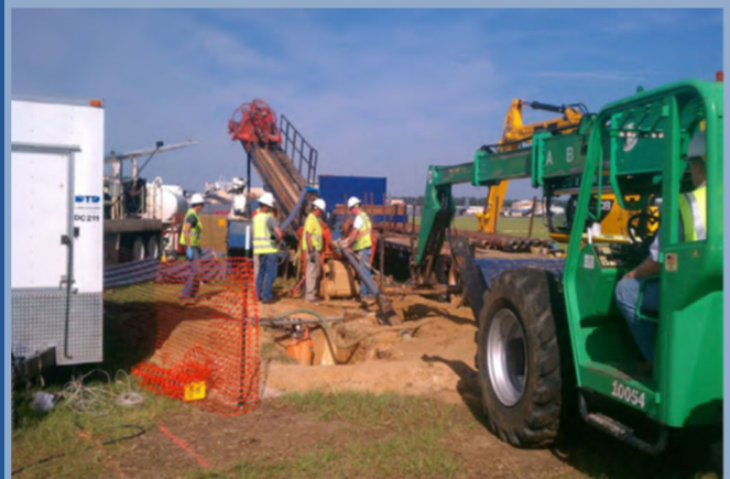
HDD Installation at SWMU 59 in 2012.
