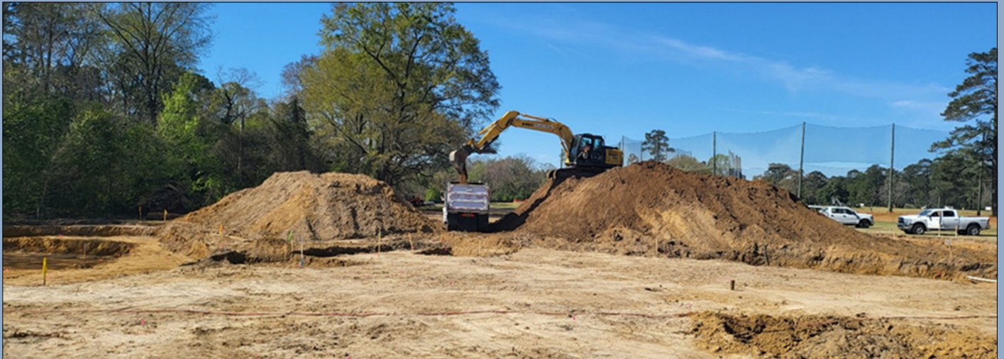
Excavation and Stockpiling Activities at TS882
